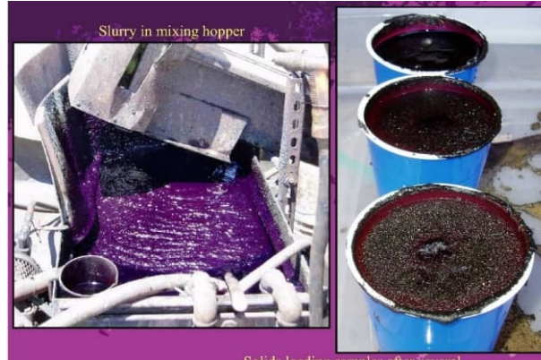
Hydraulic Slurry Emplacement
